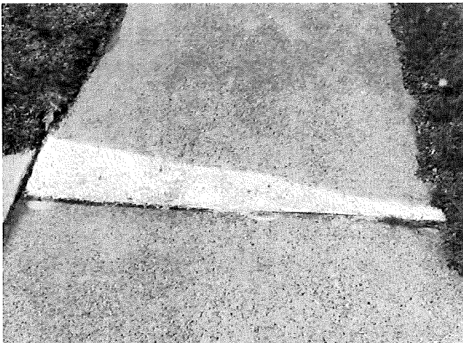
Sample Repair Photo: Defect 63 repaired on 5/1/24 at 140 10th St at 1:04 PM
