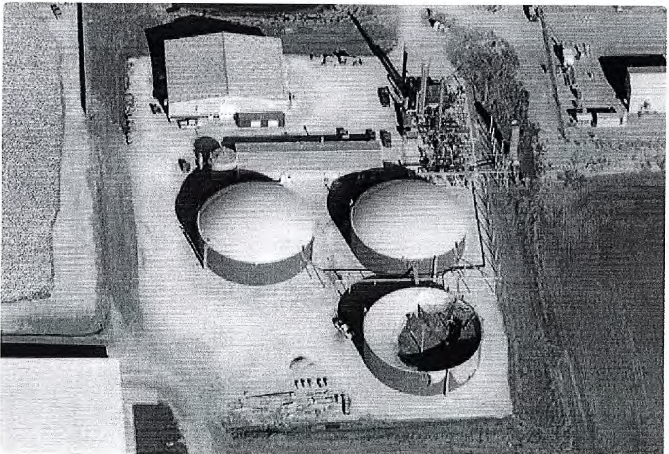
An aerial photo of the Marshall Ridge Energy Center near Story City, Iowa, Nov. 13, 2023, after a fire burned through the vinyl roof of one of the digester tanks. (Source: Beacon)
