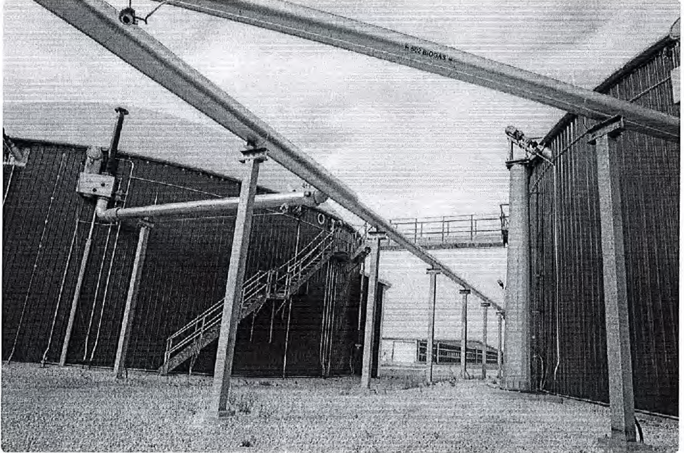
Digesters and a dairy barn are seen at the Marshall Ridge Renewable Energy Center in State Center on Sept. 18, 2024. The facility's three anaerobic manure digesters extract methane from dairy cow manure. (Nick Rohlfman/The Gazette)
