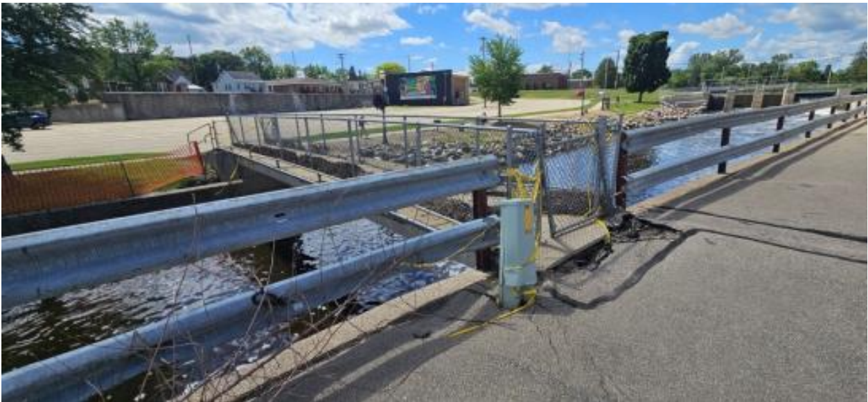
North side of Bridge Looking SW
