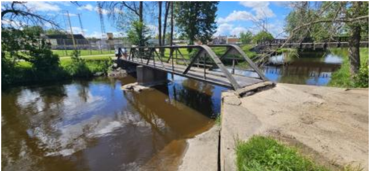
North side looking SW
