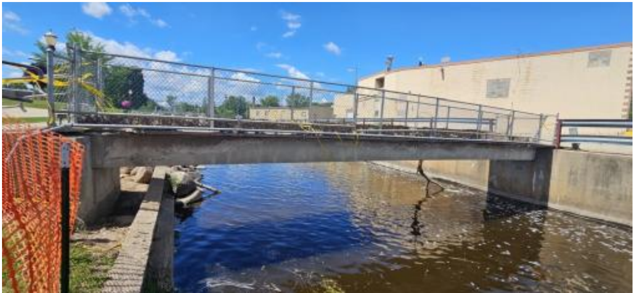
South (downstream) side of Bridge showing abutment behind retaining wall. North side rests directly on retaining wall.
