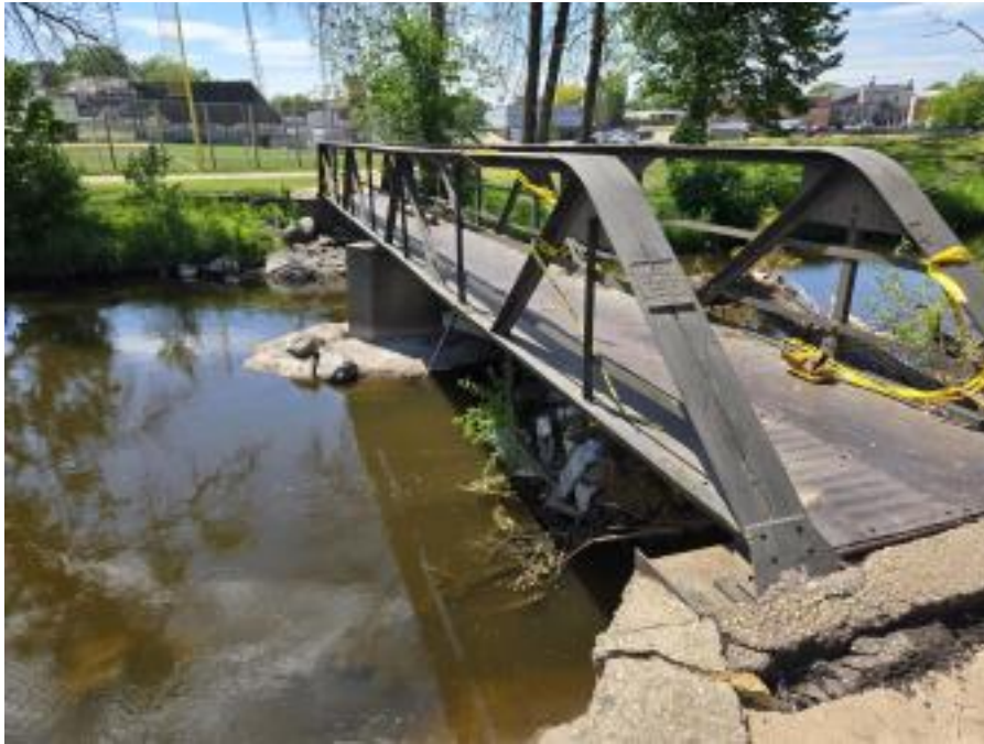
Abutments and Pier from North Side to SW
