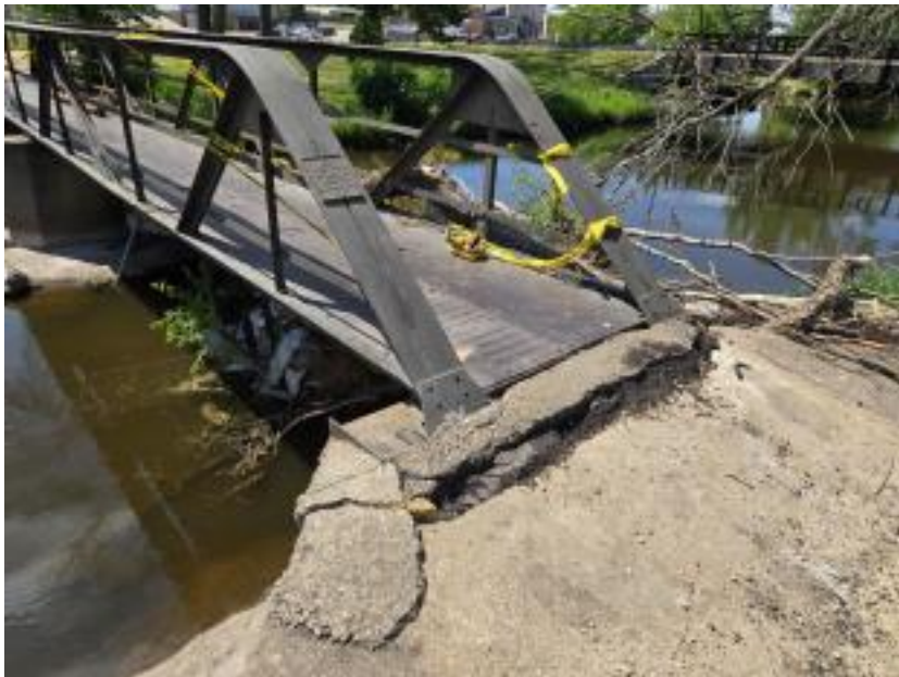
Northeast end of deck Meeting abutment
